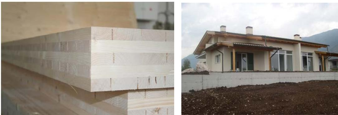
The wooden walls are covered with non-combustible insulation material and finally the building can assume any outer appearance that may be wished, just like brick houses. We should well remember that this system has nothing to do with American prefabricated houses – ordered from catalogues to get the idea – but that these are real houses, even apartment buildings adapted to the standards of European cities, solid and guaranteeing maximum thermal and acoustic insulation.
