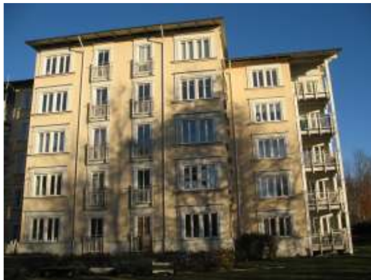
Figure 18 Light-frame 5-storey building
