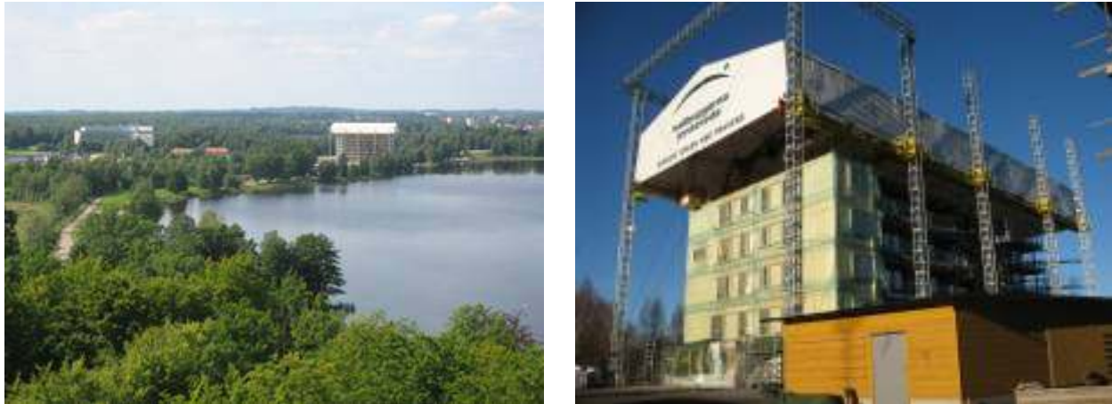
Figure 2 8-Storey building under construction
