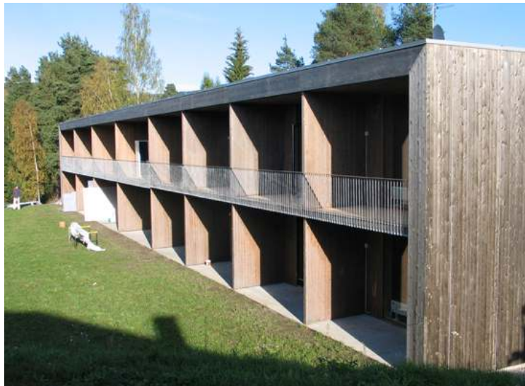
Figure 26 Concept of the 2-Storey multi-family building using wood slabs for roofs, walls and floors
