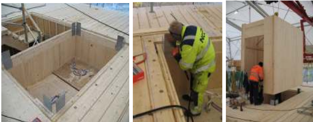
Figure 13 Connections wall-to-wall in elevator cage frame
