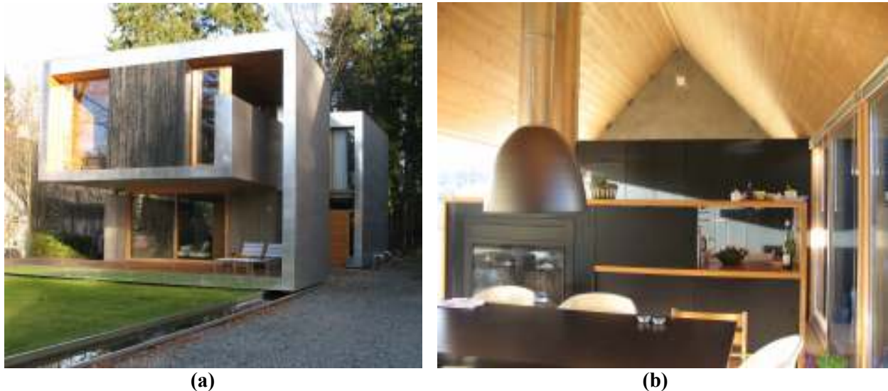
Figure 25 Single-family houses made of concrete and cross-laminated wood panels
