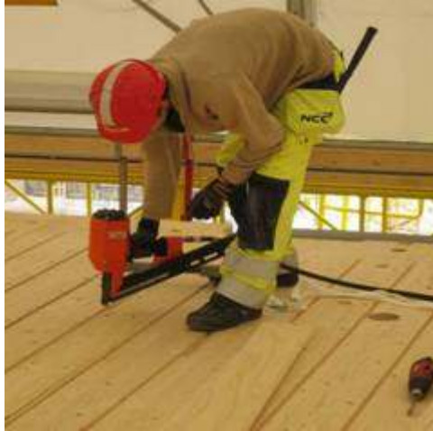
Figure 10 Connections between floor panels
