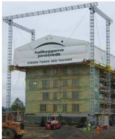
Figure 3 System of tent used during the construction
