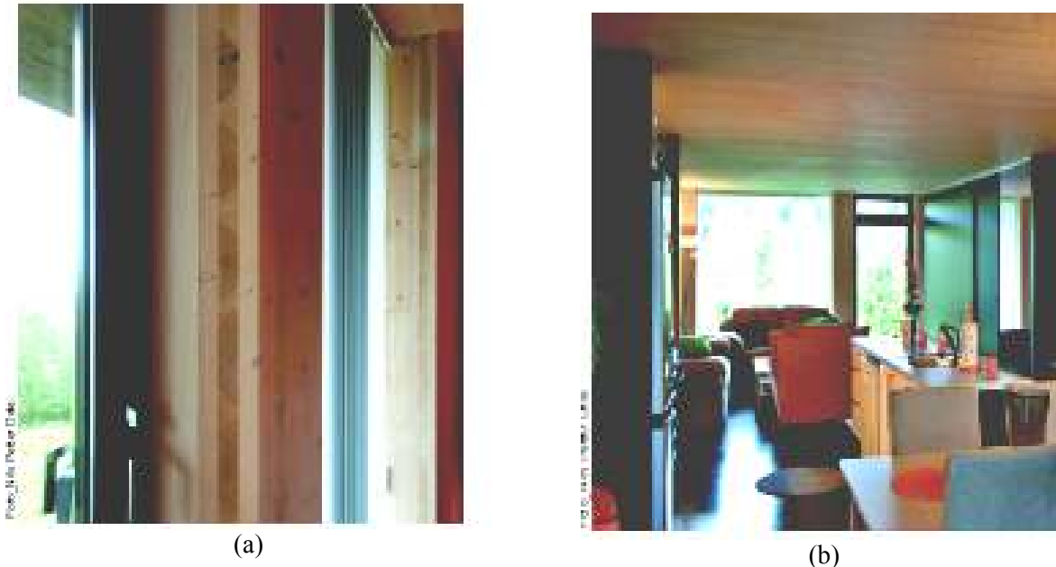
Figure 27 (a): Massive wood walls of the multi-family building; (b): Massive wood panels for ceiling and floor with topping for sound insulation
