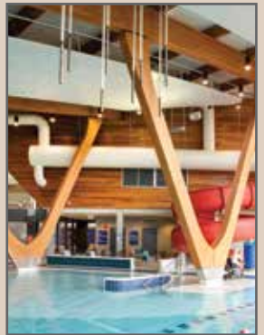
West Vancouver Aquatic Centre, West Vancouver, BC
