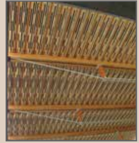
Alberni District Secondary School, Port Alberni, BC
