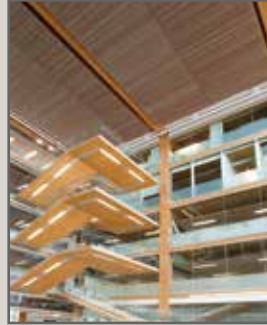
Earth Sciences Building at UBC, Vancouver, BC
