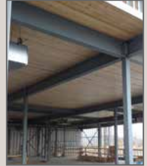
Still Creek Operations Centre, Burnaby, BC
