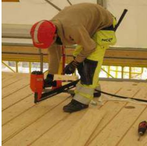
Figure 10 Connections between floor panels
