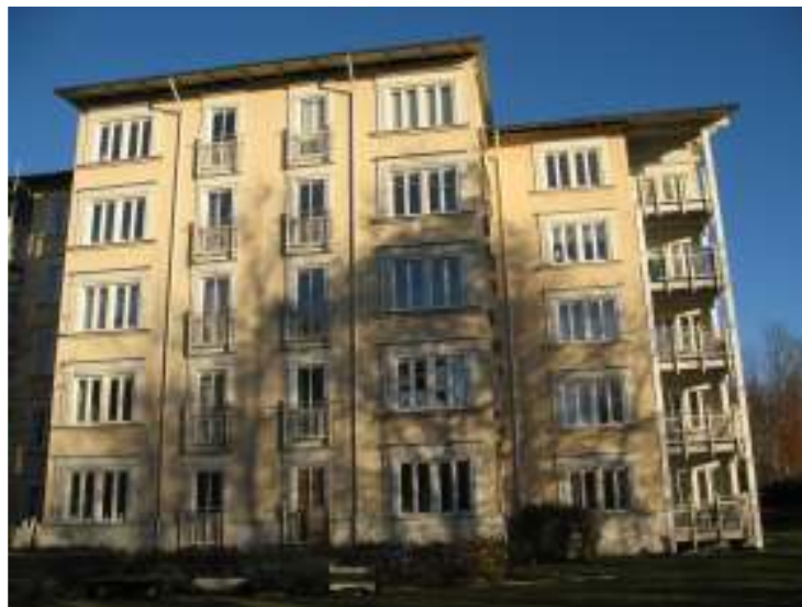
Figure 18 Light-frame 5-storey building
