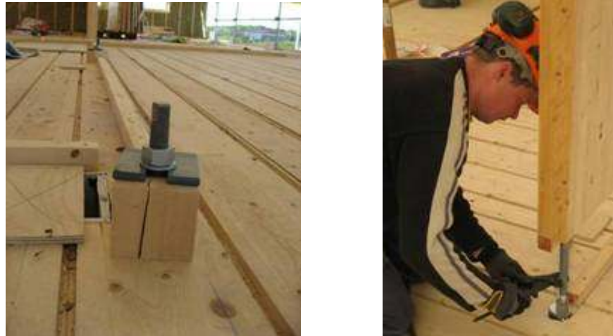
Figure 12 Connections wall-to-wall for lateral load resisting system
