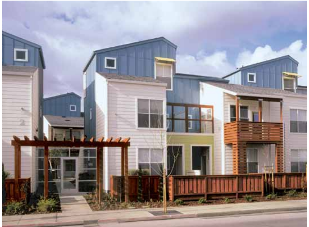
PHOTO 1: Wood-frame construction produces high quality and affordable housing.
