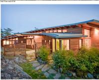
The building is off all energy grids and is oriented to maximize solar gain. Its central spaces are transparent so that the southern sun penetrates deeply into interior spaces, warming floors and walls. Ocean views to the south and west are open to all spaces including the south-facing outdoor room and terraces
