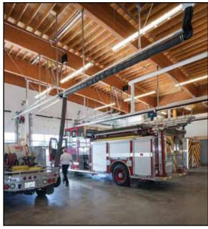
"Interesting to have the joists sit on the glulam, allowing the light to filter through."
