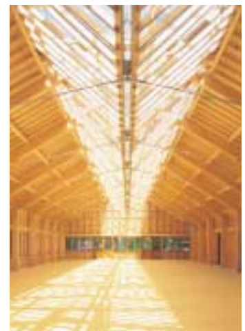
MOORELANDS CAMP DINING HALL LAKE KAWAGAMA, DOSET, ONTARIO PHOTOS: JAMES DOW ARCHITECT: SHIM-SUTCLIFFE ARCHITECTS
