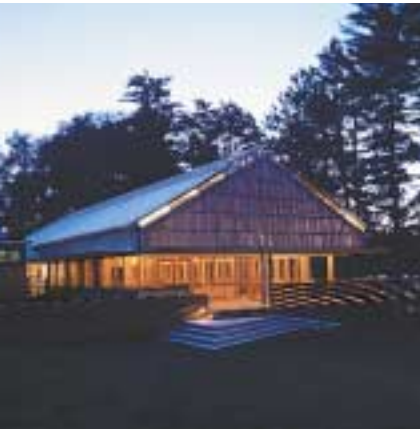
MOORELANDS CAMP DINING HALL LAKE KAWAGAMA, DOSET, ONTARIO PHOTOS: JAMES DOW ARCHITECT: SHIM-SUTCLIFFE ARCHITECTS
