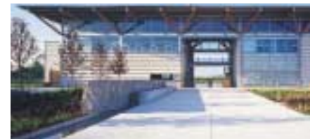
JACKSON-TRIGGS NIAGARA ESTATE WINERY NIAGARA-ON-THE-LAKE, ONTARIO PHOTOS: PETER A. SELLAR/KLIK AND DESIGN ARCHIVE/ROBERT BURLEY ARCHITECT: KUWABARA PAYNE MCKENNA BLUMBERG ARCHITECTS
