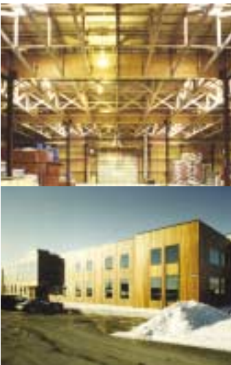
ROCKET LUMBER WAREHOUSE/OFFICE BUILDING MISSISSAUGA, ONTARIO PHOTOS: PEDRO HO ARCHITECT: ALLAN RAE, ARCHITECT
