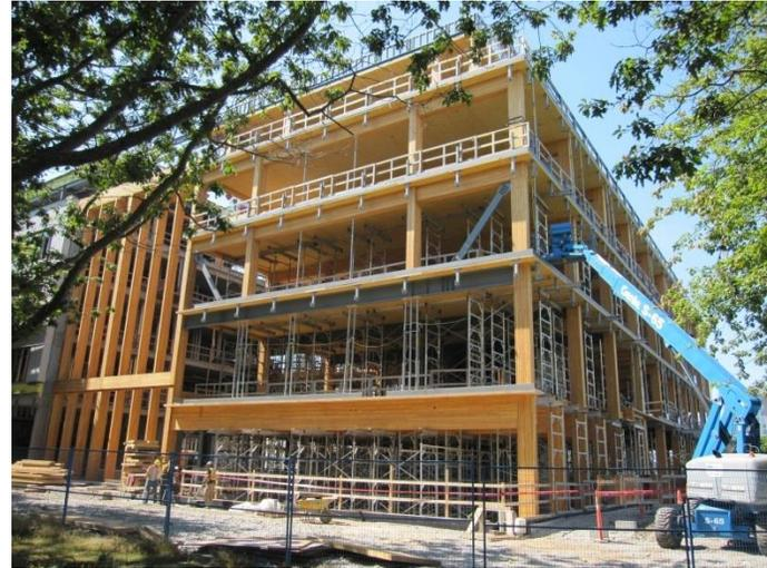
Photo of the Earth Science Building north wing, a 5 storey heavy timber structure, under construction.
