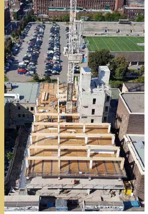
Bird's-eye view of 80 Atlantic during the installation of the timber columns and beams for the third floor.
