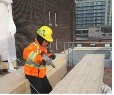
Carpenter uses 600 mm screws to stitch together two pieces of glulam to complete the assembly of a beam prior to its installation.
