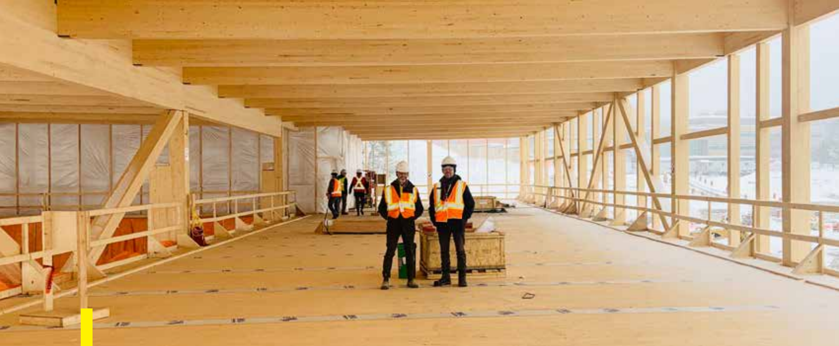
Figure 11. Mass Timber Construction
