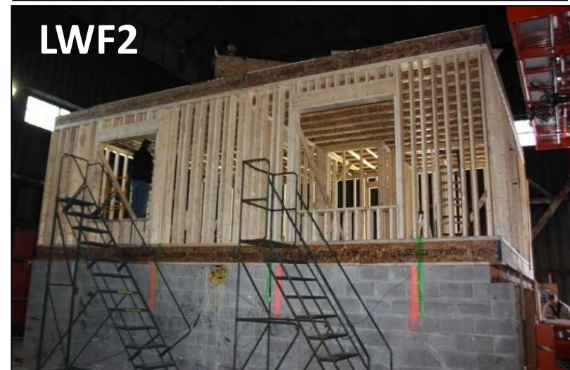
Figure 29. Large-scale apartment test structures under construction.
